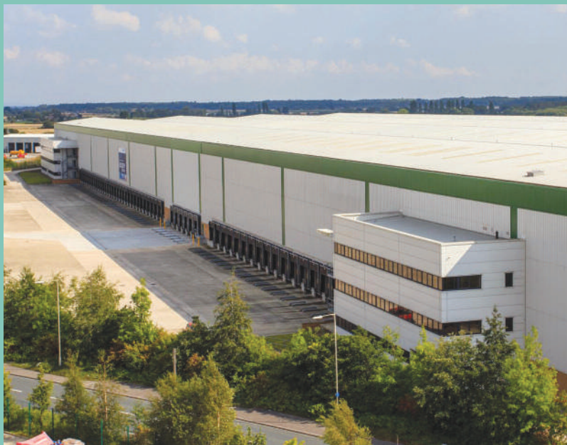
Legal & General facility at Sherburn-in-Elmet, North Yorkshire
