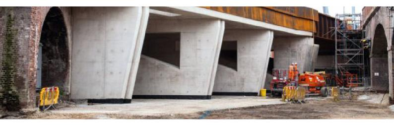
Whereas a traditional concrete requires anywhere up to 28 days to reach full strength, high-early-strength concrete can achieve this in just 48 hours. This therefore helps speed up project delivery and improves efficiency by enabling the next phase of construction to commence sooner. Tarmac's readymix business manager, James Macintosh, explains:
