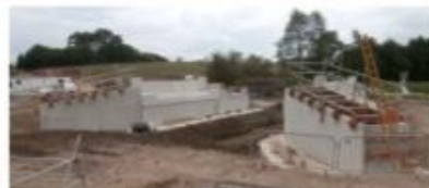
Figure 1: Modular construction on Stafford Area Improvements Project (Laing O'Rourke)
