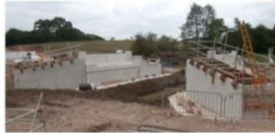
Figure 1: Modular construction on Stafford Area Improvements Project (Laing O'Rourke)
