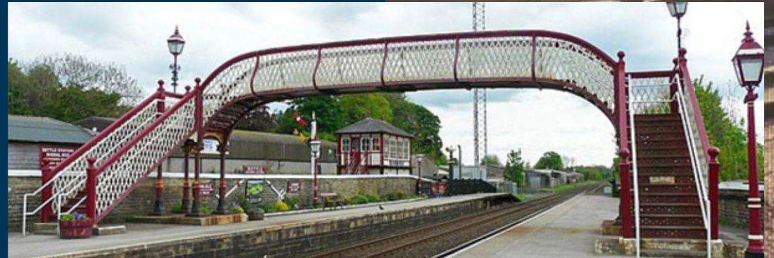
Settle Station Footbridge
