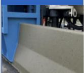
Slipform Concrete Barrier
